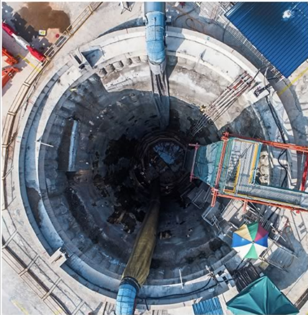
The intervention shaft, which required excavation using controlled blasting to mine shafts which go down as deep as 60m. An access point for tunnel maintenance, there are three escape and ventilation shafts each along the MRT2 alignment.
