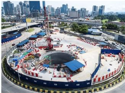
The intervention shaft, which required excavation using controlled blasting to mine shafts which go down as deep as 60m. An access point for tunnel maintenance, there are three escape and ventilation shafts each along the MRT2 alignment.
