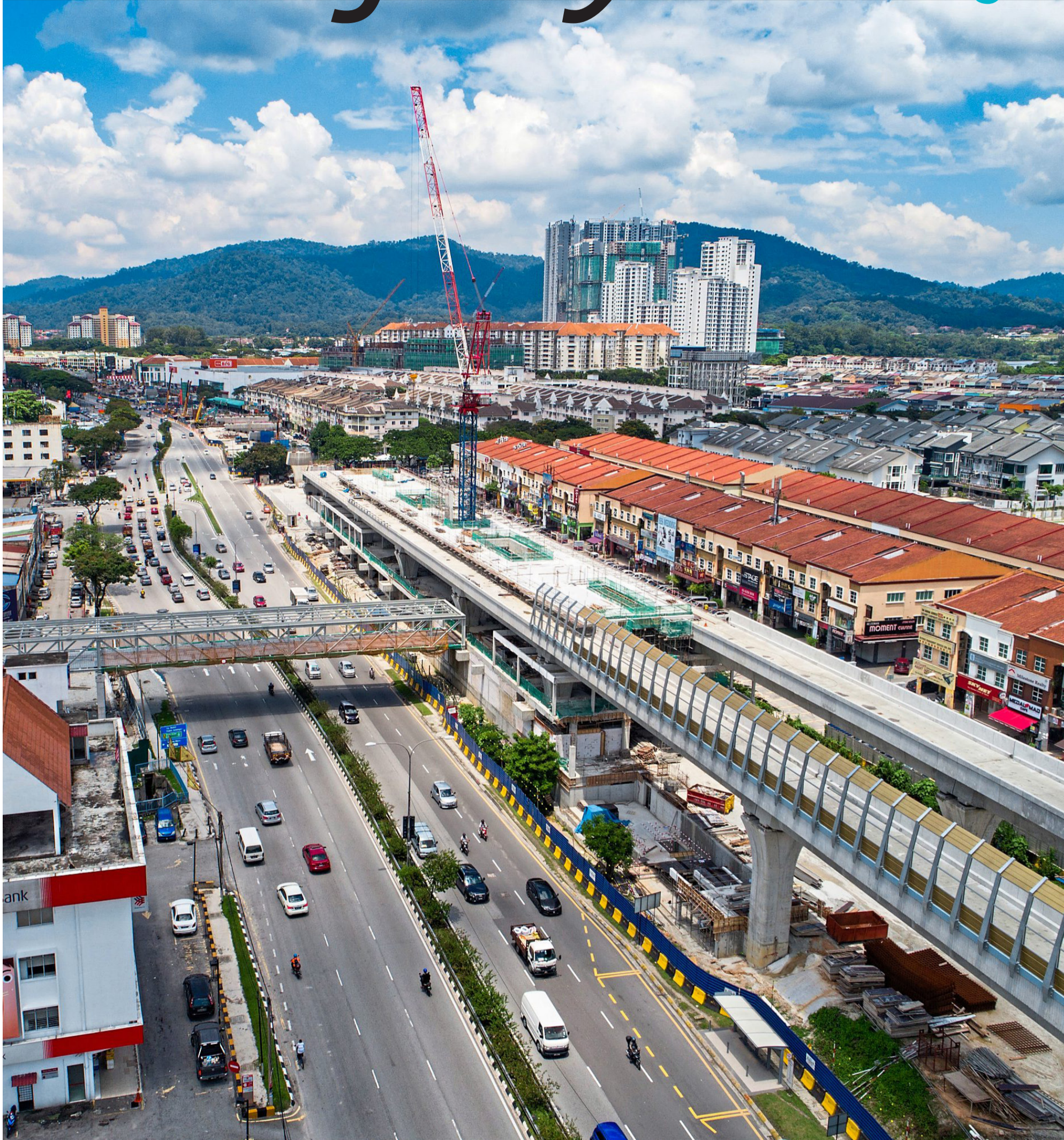
The civil and structure works of the MRT Kepong Baru station are near completion. This station on the SSP Line is 60% complete with ongoing progress on systems, mechanical and electrical works, and architectural finishing.
